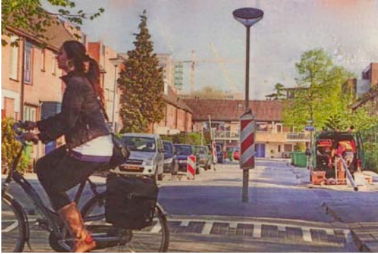
Figure 3: Street light installed at the center of the intersection
