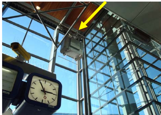
Figure 2: Bijlmer station trolley enclosed by support beam.
